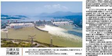
三峡大坝开闸泄洪
